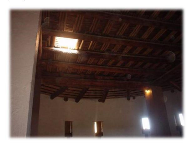
Photo 35: The roof of the Great Kiva weighed 95 tons and was one of the engineering feats of the Anasazi, Aztec, New Mexico.
