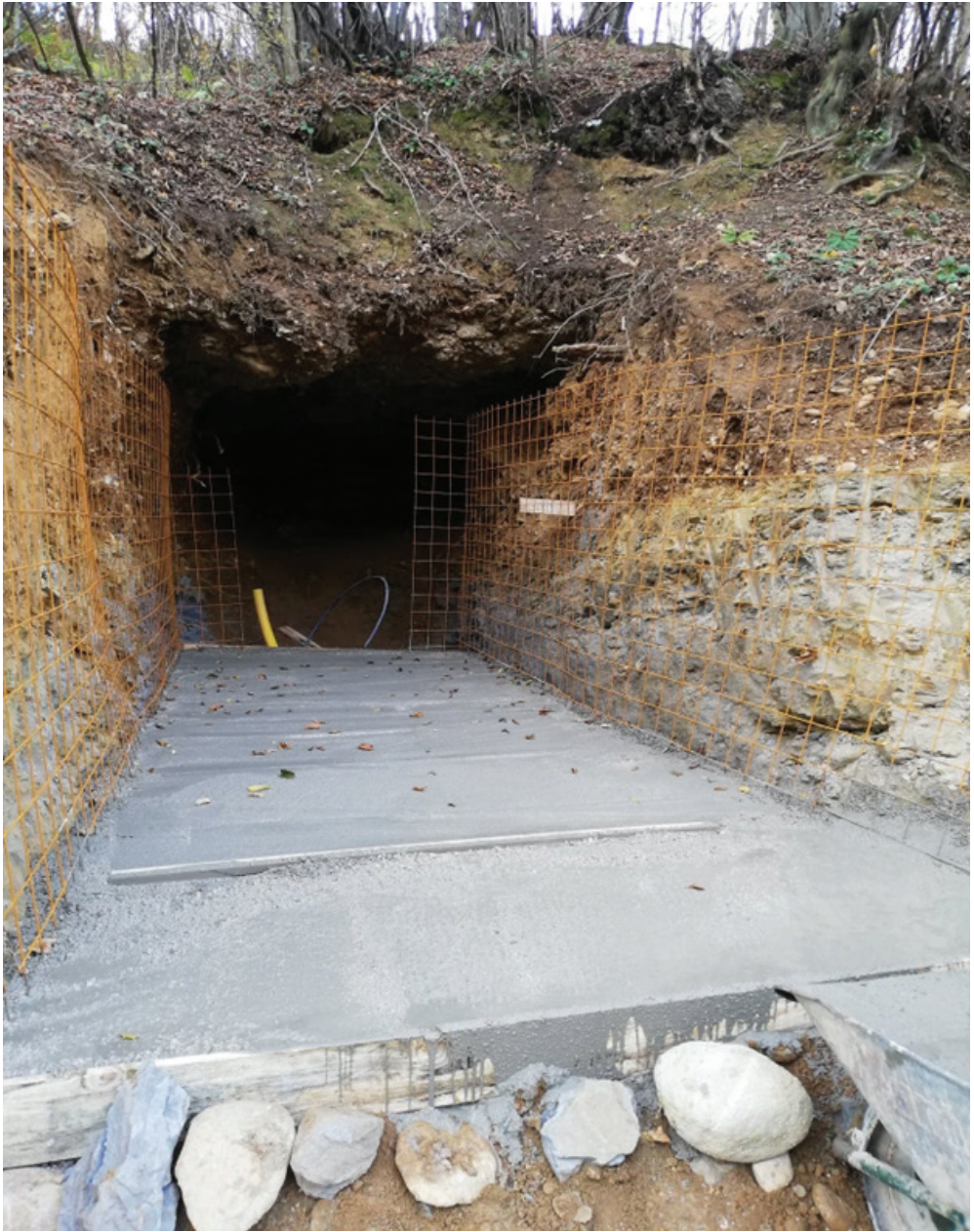
Figure 14: Preparation and protection the entrance of Ravne 4 tunnels, 2019 (photo: A. Agić)
