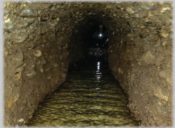
This flooded section is over 50m long and its dimensions are h.110cm x w.100cm. Some water droplets, when percolating through the conglomerate, may split apart upon impact with the surface of the rocks. This agitation causes the droplets to lose electrons and become positive ions. The surrounding oxygen may absorb those electrons and become negative ions. This phenomenon is known as the 'Lenard Effect' and may explain the high concentration of negative ions within the tunnels.
