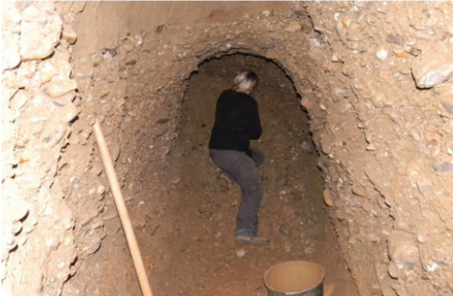
Photo 7; Ravne Tunnels being excavated in 2010. Loose rubble material is being removed from the blocked passage.
