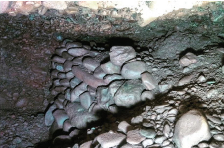
Photo 60; Drywall in Ravne4 discovered with loose rubble behind it
