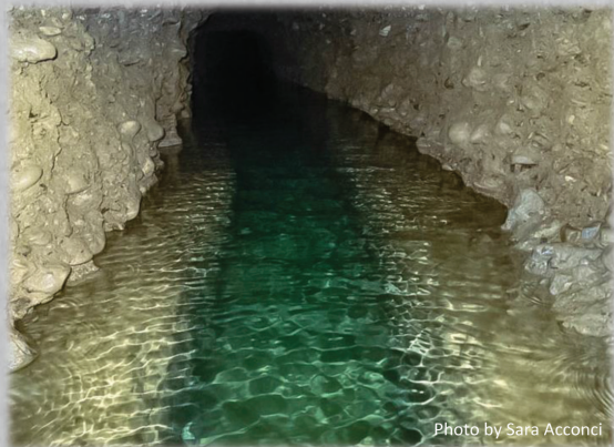
The above photo shows part of the longest water tunnel section, which runs southeast for almost 200m. It can be seen that this passage has been channelized along its centreline. This open section of tunnels was first accessed and explored towards the closing of 2010 when excavations reached the meeting point of several passages, now named the 'Water Tunnels Chamber'.
