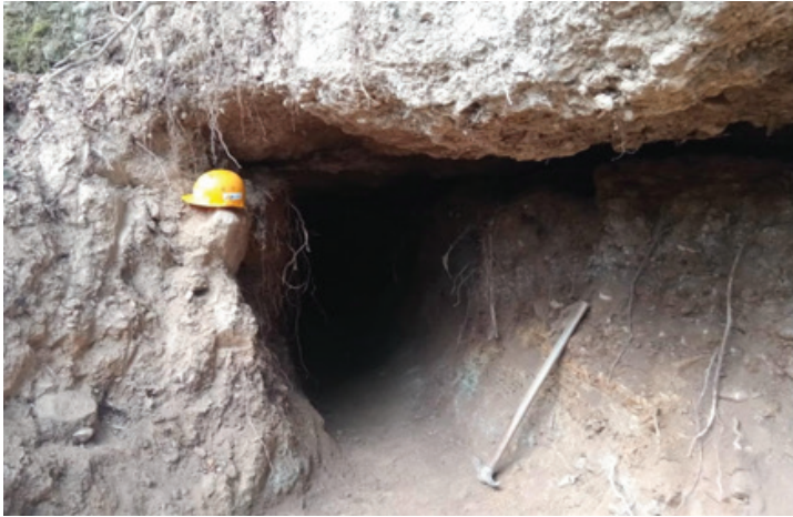
Photo 23; Cavity 'C3' after excavating to 8m tunnel depth. Passage seen cutting down into underlying marl beds. Tunnel height is approximately 1.7 m and 1.5 m wide
