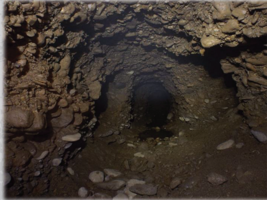
Photo above shows the 23m long northwest heading passage, connecting chambers R4-1 & R4-2. Two side tunnels without drywalls, left and right, can also be identified within this image. Both of these side tunnels are blocked with loose rubble material in the same manor as minor passages across the Ravne Tunnels Complex.
