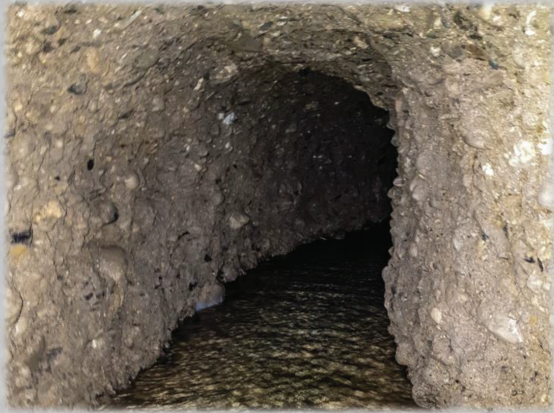
One of the flooded water sections of the Ravne Tunnels. This water section is south of the 'blue lake'. The placid water is captured within the tunnels due to the underlying geological layers being impermeable. The water contained within the Ravne Tunnels has slowly permeated through the surrounding conglomerate rock, which contains fine carbonaceous clays, sands and pebbles. These materials filter out impurities from the water, leaving it crystal clear and perfectly fit for human consumption.
