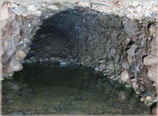
Above is a small widened chamber containing captured water, named 'Blue Lake'. It measures /.5m x w.1.6m. Towards the rear of the chamber is a passage infilled with loose, unconsolidated rubble. This blocked passage will connect with one of the infilled side tunnels located along the thoroughfare heading southeast, north of the 'Blue Lake'.
