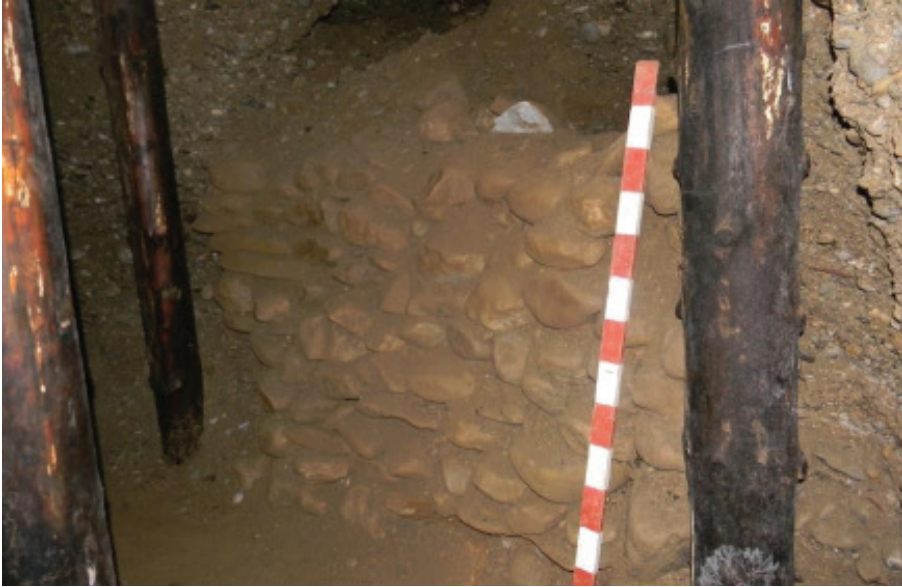
Photo 5; One of over 50 drywall constructions within the Ravne Tunnels. Drywalls mark position of infilled side-tunnels.
