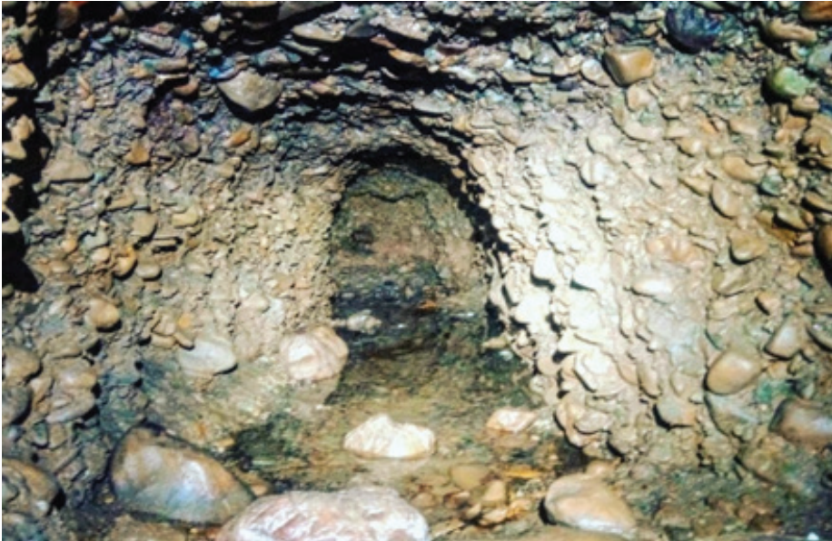
Photo 59; A small emptied passageway in Ravne4 heading in a south- westerly direction. Water accumulates on the floor of the tunnel.
