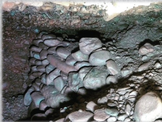
Photo above shows the first and only fully intact drywall so far identified within the explored sections of Ravne4. The presence of drywalls within Ravne, Ravne3 and Ravne4 infers all are part of the same tunnel network, and may have at one time all been physically connected. Within the centre of the drywall is a flat faced slab, one of the small design cues noted previously on some of the drywalls within the Ravne Tunnels.
