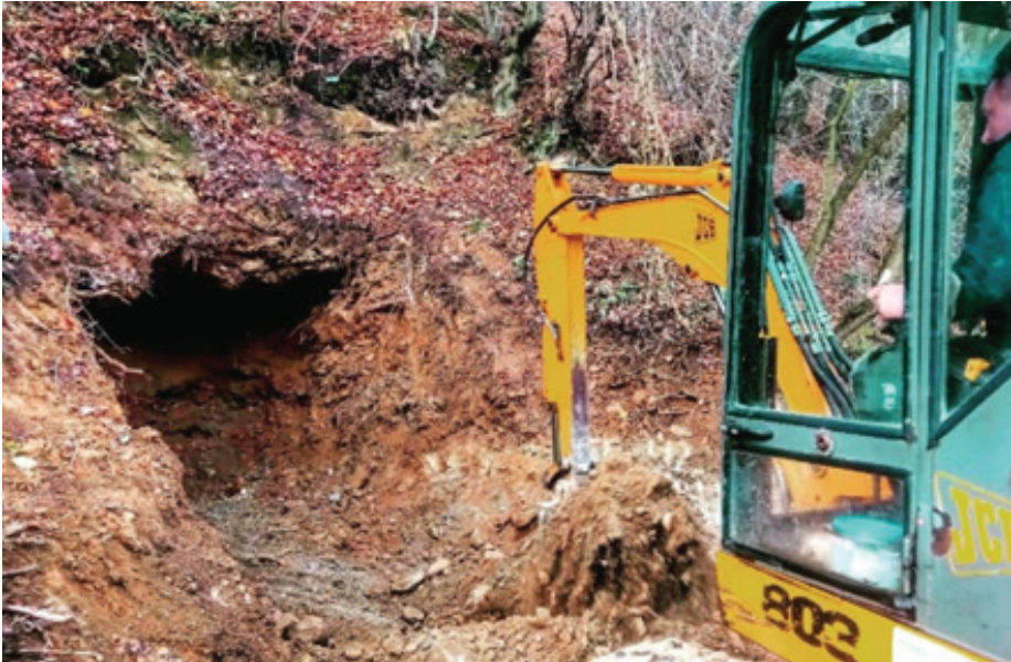
Photo 57; November 4, 2019. Ravne 4 entrance is being cleared shortly after its discovery.
