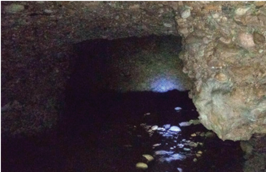
Photo 24; At 8m tunnel depth a section of passages with chambers free from rubble infill was found, allowing free movement within the cavity.
