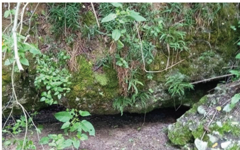
Photo 8; Cavity opening Ravne3 'C2' before excavations. Gap between floor and base of conglomerate is approximately 15-20 cm. Cold streams of air exiting the small cavity hinted at a larger cavity space allowing air circulation.
